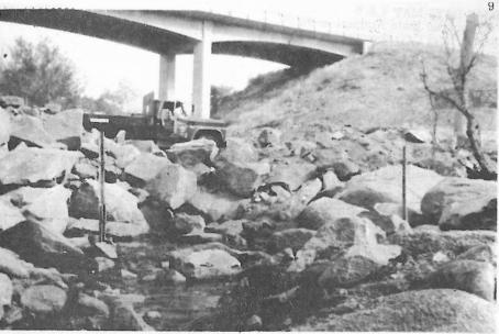
This shows effect of big blast as prepared in photos on preceding pages: hard blue granite is split asunder and tossed into creek which runs year around under Willows bridge. This will be the foundation for access road south of freeway.
