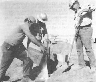
Here's how blasters handle harmless explosive, pouring grains into holes in granite which is ignited by stick of dynamite from fused cap. This explosive is a fertilizer, but when mixed with distillate it becomes a powerful blasting compound. is far safer to handle than other materials. This at the Willows. See photo next page.
